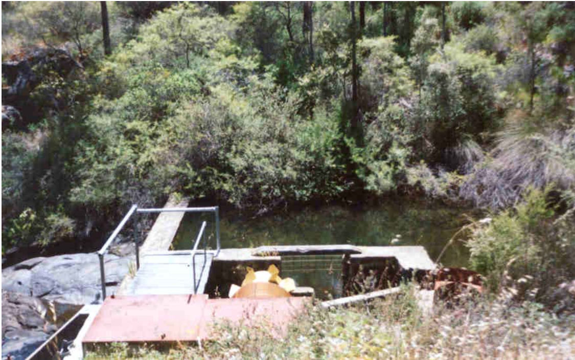
Photograph 1 - Existing Pipehead Weir
