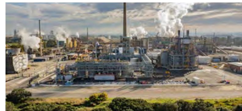
Industry operating at the Western Trade Coast. Credit: BHP Nickel West.
