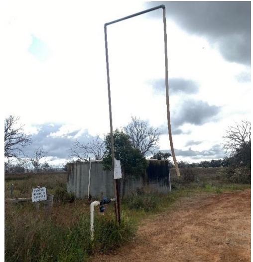
Tank and standpipe
