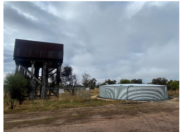
Water tank at Kylie Siding
