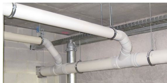
Photo 2: Connection of branches using unequal 45° junctions
