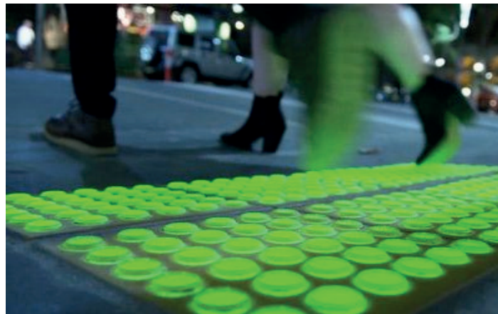
Image Four, Melbourne In-Ground Traffic Light
