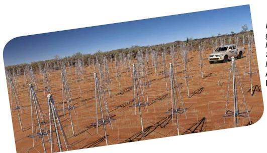
Image left: A computergenerated image of what the low frequency antennas of the Square Kilometre Array will look like. (Credit Swinburne Astronomy Productions/ ICRAR/U. Cambridge/ASTRON)
