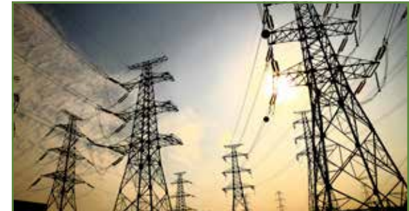
A retail electricity CUA has made it easier for agencies to reduce their electricity costs
