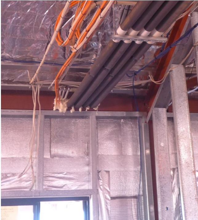
Figure 27 Group multiple service lines and treat as a single penetration. Use adhesive tape to seal services to the vapour barrier and expanding foam to fill gaps on the inside face of the penetration.
