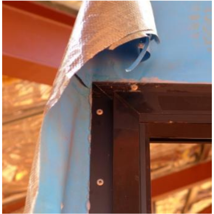
Figure 26 Provide a margin around window penetrations to allow vapour barrier to be sealed against it
