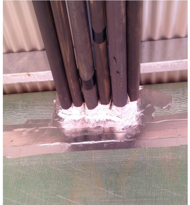
Figure 27 Group multiple service lines and treat as a single penetration. Use adhesive tape to seal services to the vapour barrier and expanding foam to fill gaps on the inside face of the penetration.
