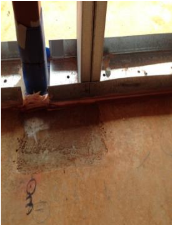
Figure 29 To increase the tightness of the vapour barrier, seal inside of bottom plate to floor before installing wall linings
