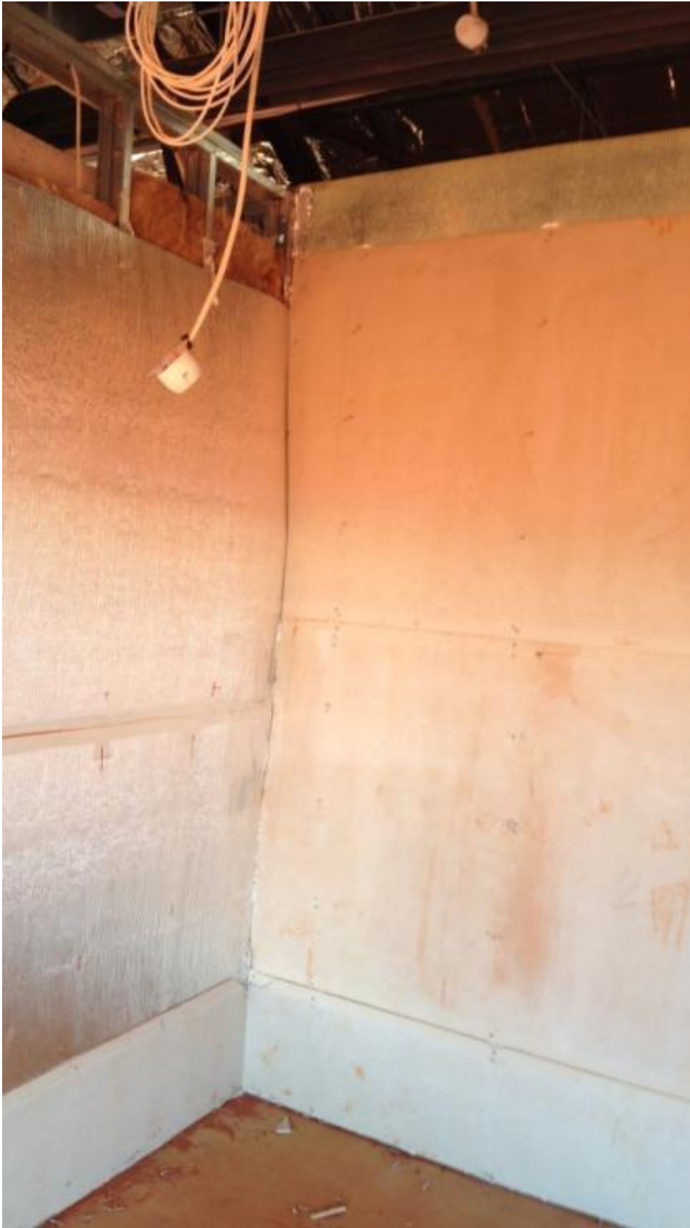
Figure 25 Install a vapour barrier to internal walls to separate conditioned from non-conditioned spaces. Vapour barrier to be located on non-conditioned side of the wall.
