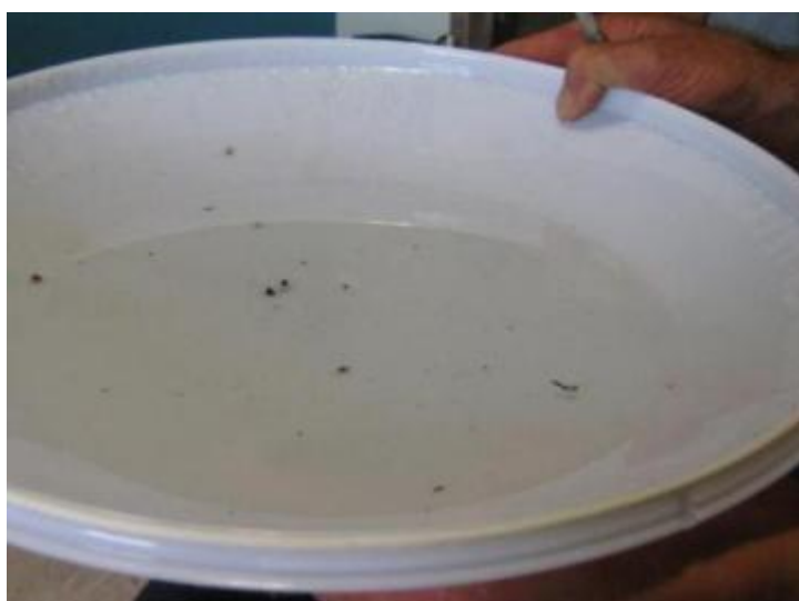
Figure 14 Moisture trapped inside light fittings is a dangerous consequence of condensation
