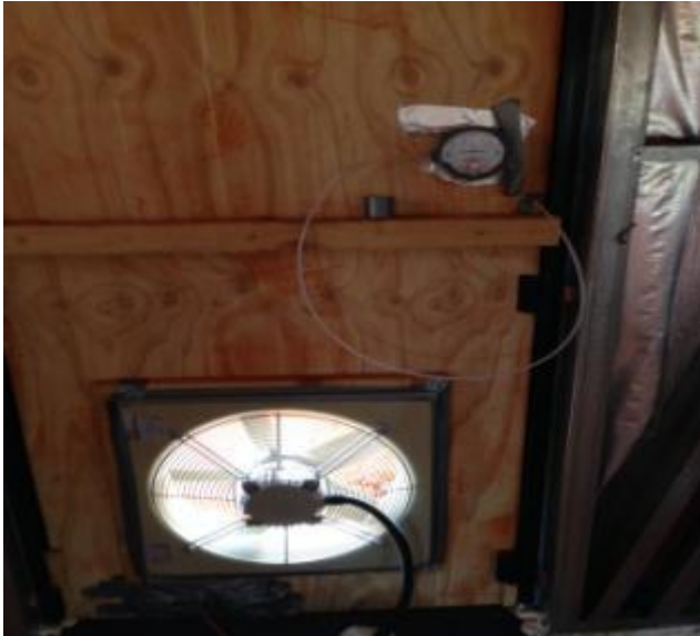
Figure 32 Increase fan speed until the pressure inside the building is 10 Pa above the outside pressure and measure the air flow from the fan using a certified hood.
