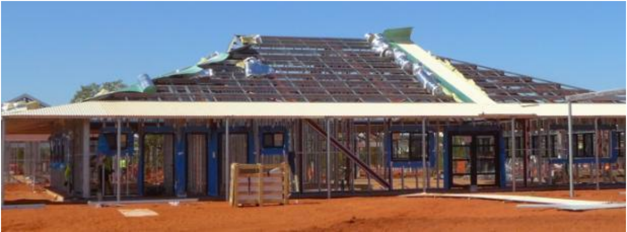
Figure 20 Provide vapour barrier behind all roof cladding.
