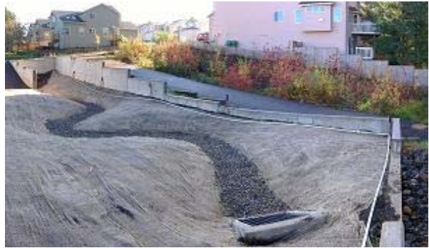
Figure 2: Two bio-swales for a housing development. The one in the foreground is under construction, while the one in the background is already established.
