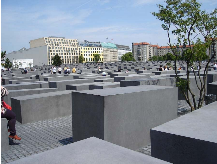
Figure 4: An anti-graffiti coating has been used to protect all the concrete 'plinths' of the Holocaust Memorial in Berlin
