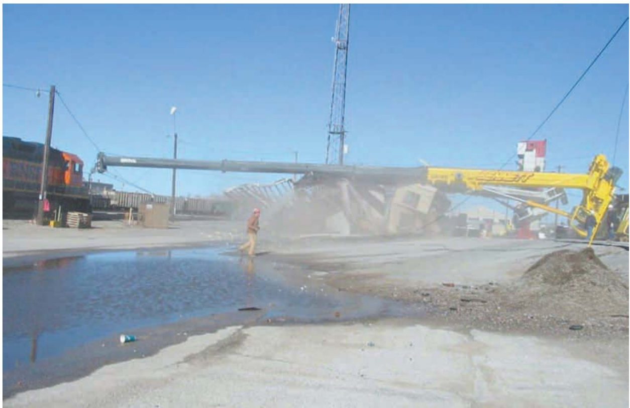
Crane overturned across rail reserve.
