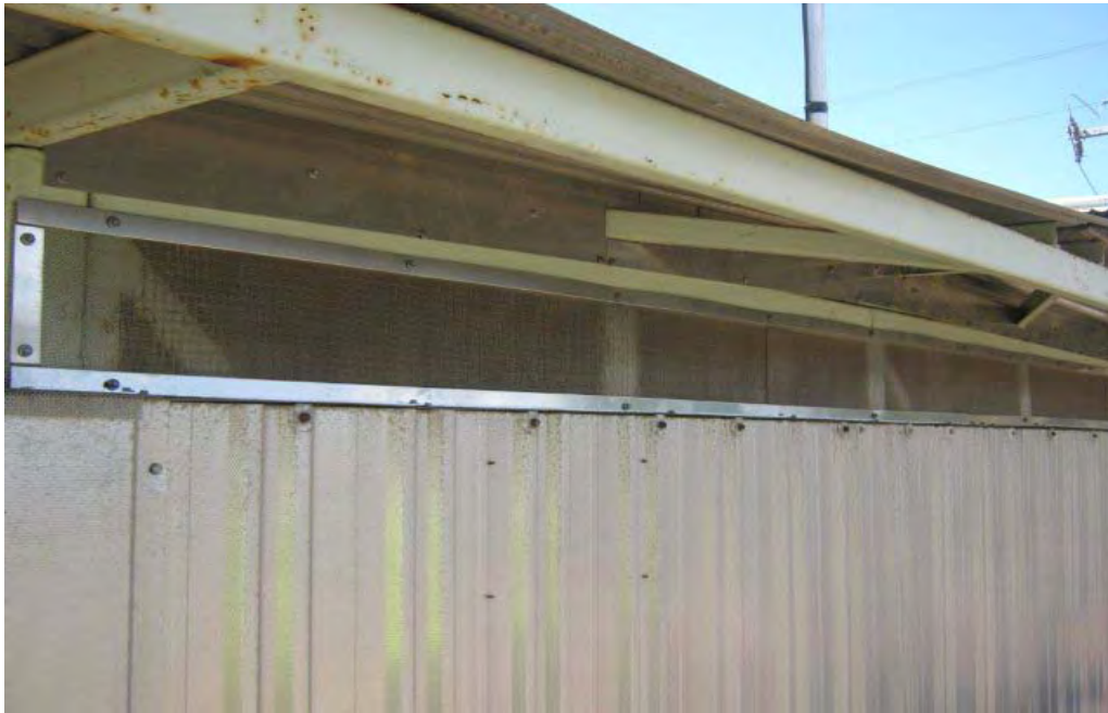
Photo 3 - Scott Road Pump Station post-fire, taken on 15 February 2011 (including visible mitigation works undertaken prior to fire)
