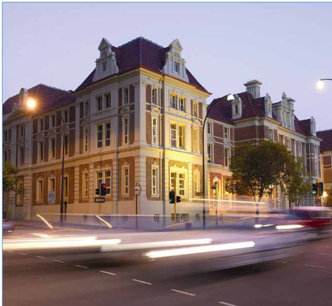
Old Treasury Building
