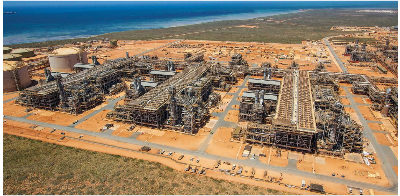
Gorgon gas processing trains. Photo: Chevron
