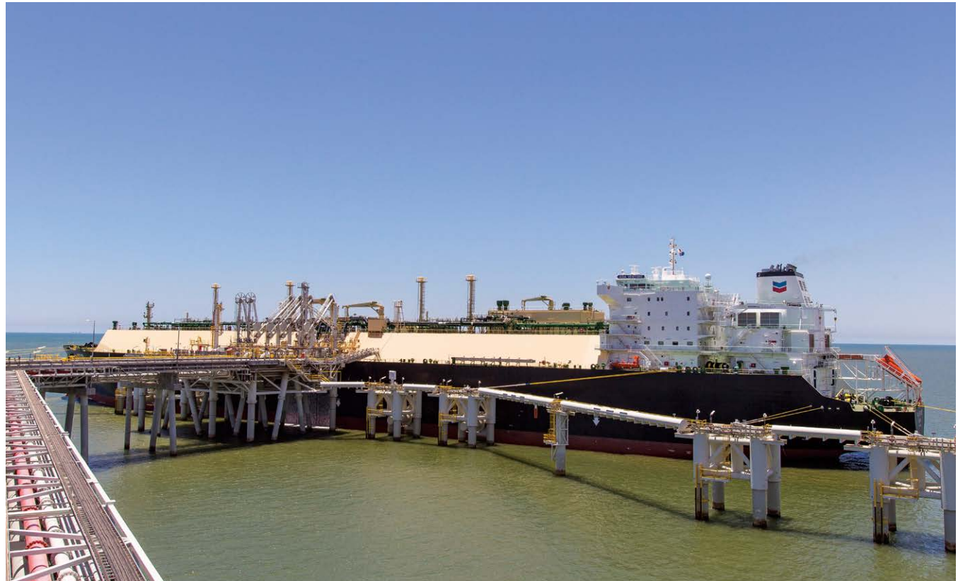
First Chevron Wheatstone LNG cargo is loaded. Photo: Chevron
