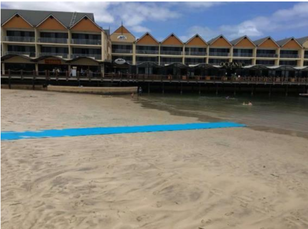
Figure 16 Access improvements at Swimmer's Beach, Keith Holmes Reserve, Mandurah
