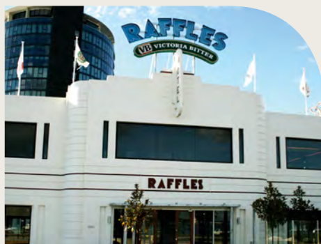
LEFT: Former Midland Railway Workshops flanging workshop now the WA Police Operations Support Facility (Traffic Operations); Raffles Hotel, Applecross
