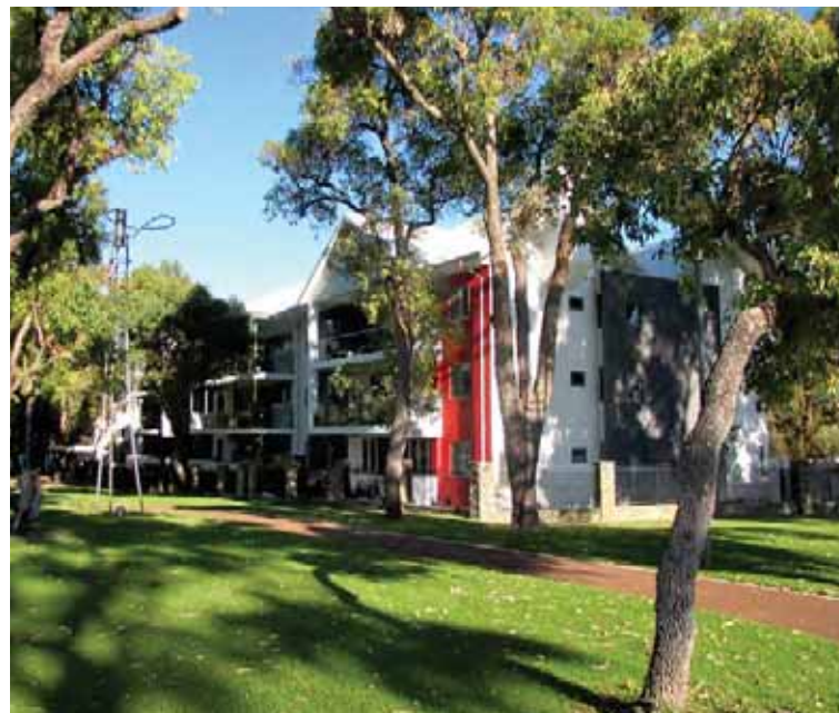
Reduced rear setbacks and large balconies strengthen the connection between apartments and adjoining parkland while also providing passive surveillance. Building footprint is 50m x 20m deep (Block: 65m x 35m). Churchlands, WA.
