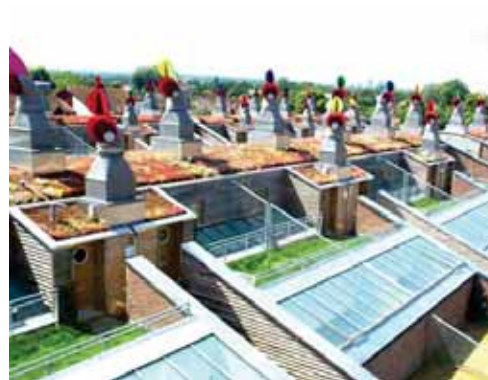
Thermal stack ventilation exhausts provide a design feature in the Bedzed development in London.
