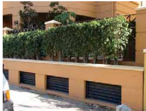
Ventilation for semi-basement parking provides space for street planting.
