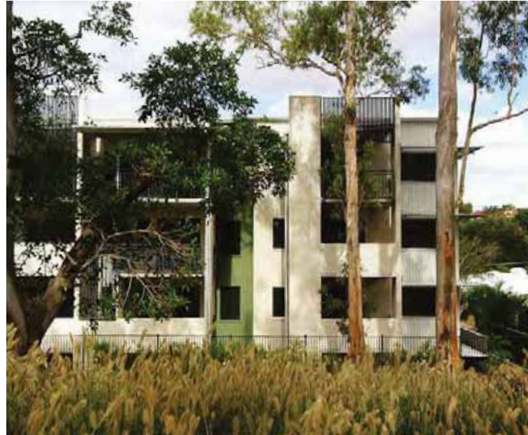
Affordable Housing with a strong focus on providing communal spaces for occupants Industrial materials have been utilised, with unfinished concrete block construction combined with steel balustrades, rafters and wide pan sheeting. Kelvin Grove, QLD
