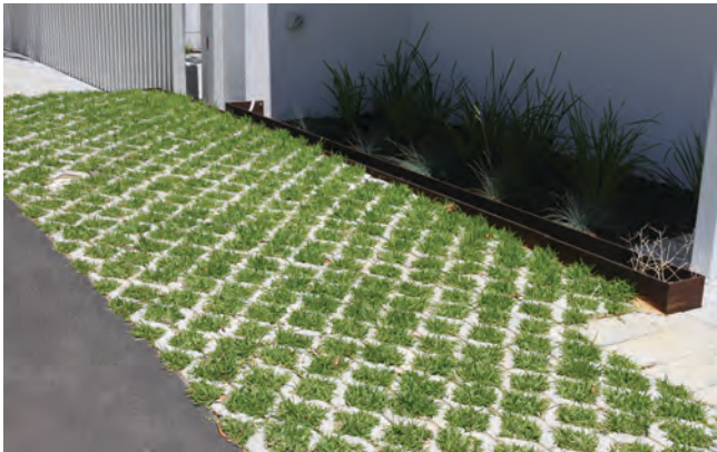
Photo G2.3d Permeable pavers planted with hardy waterwise plants can provide trafficable areas
