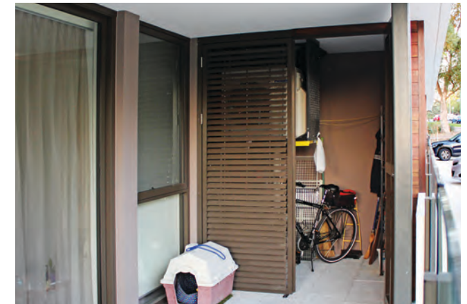
Photo G3.5a and b This storage area has been neatly integrated into the design of the balcony, is conveniently located, of useful size and proportions, weatherproof, and screened from view
