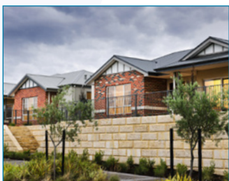
Attached houses, The Vale - R40 Image courtesy of APG builders
