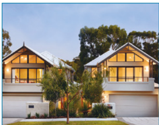
Traditional houses on narrow lots, Watermans Bay - R20. Image courtesy of WBN builders
