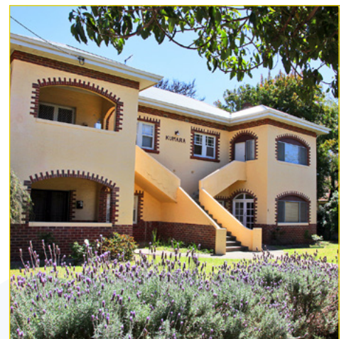
An example of a traditional maisonette building in Nedlands.
