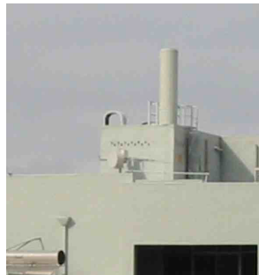
Antenna disguised as a chimney
