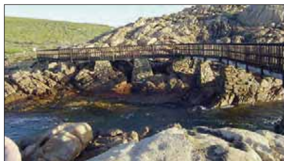
Image 29: This walkway at Canal Rocks, Yallingup, blends with its setting as the colour of the timber matches that of the rock base and natural stone has been used for foundations.
