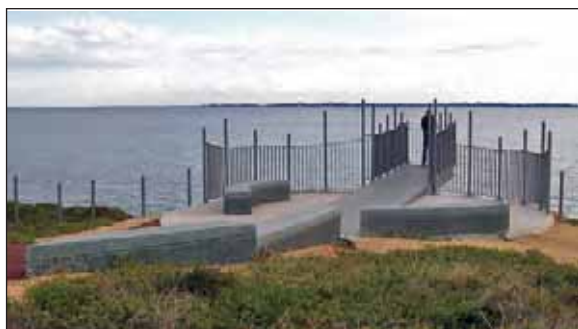
Image 77: The design of this coastal lookout at Naval Base reflects its industrial setting.
