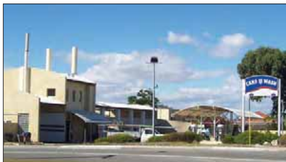
Image 102: This car wash in Doubleview has effectively camouflaged the mobile phone structures on the top of the building.
