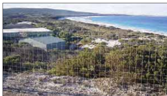
Image 25: Aquaculture development at Bremer Bay located in a swale behind the foredune where it is not visible from the beach.
