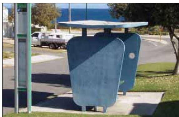
Image 79: The colouring of this City Beach bus shelter is a reminder of its coastal setting.
