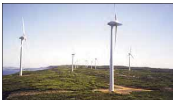
Image 100: Sand Patch wind farm (Albany) displays minimal clearing at the base of the turbines.
