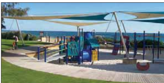
Image 50: Play equipment can create visual clutter in foreshore reserves unless it is carefully designed, as in this example at City Beach. Here the colours match the coastal setting, the equipment is placed below the natural ground surface and the overall design is of a high quality.
