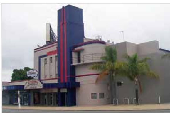
Image 103: The art-deco Windsor Theatre in Nedlands is another good example of effective camouflage of mobile phone towers. Equipment is located within a false extension to the tower.
