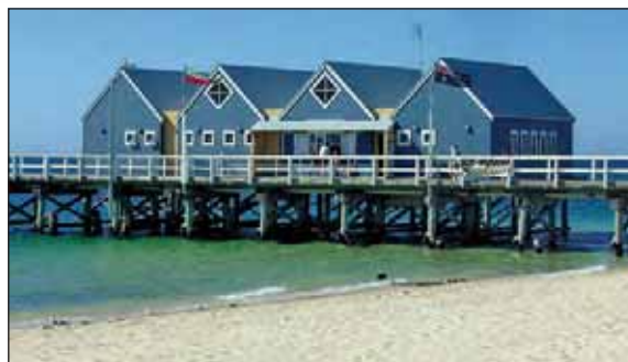
Image 33: This building at Busselton jetty is prominent due to its location however its colour and form link it to the natural and cultural elements of its setting: the coastal landscape and historic jetty.
