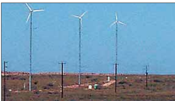
Image 95: Turbines located in flatter terrain.
