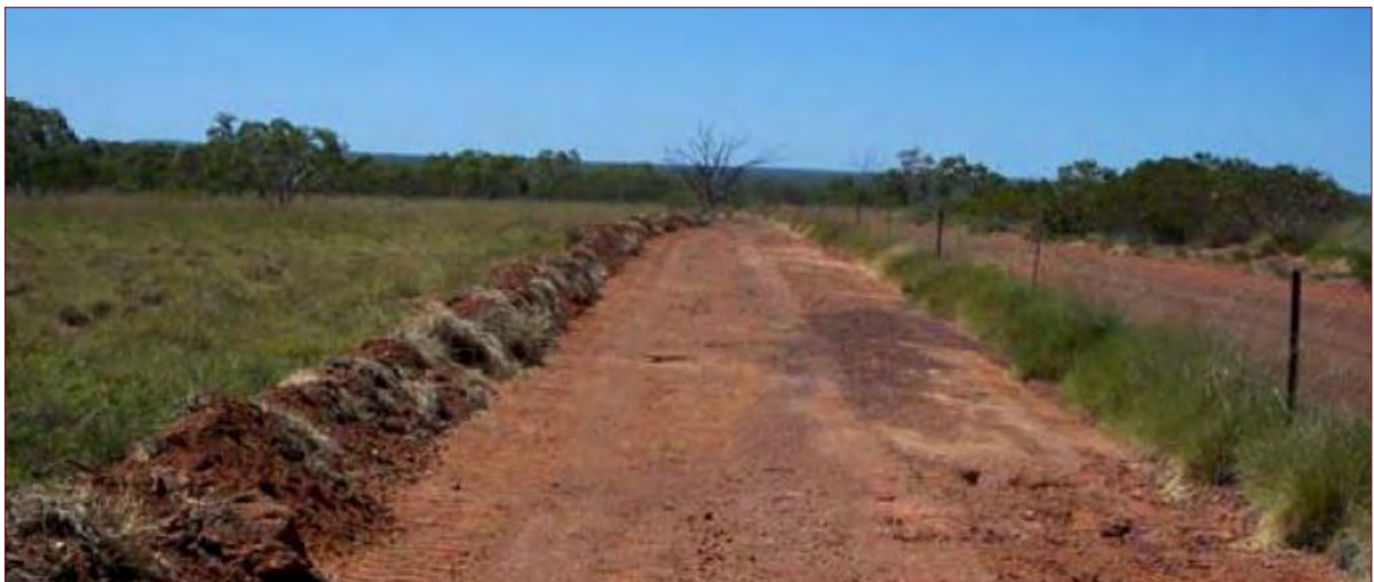
Figure 23: Freshly graded track with prominent windrow
