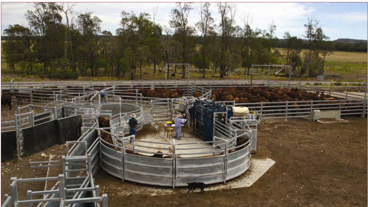
Figure 39: Cattle yard incorporating design elements for low-stress stock handling
