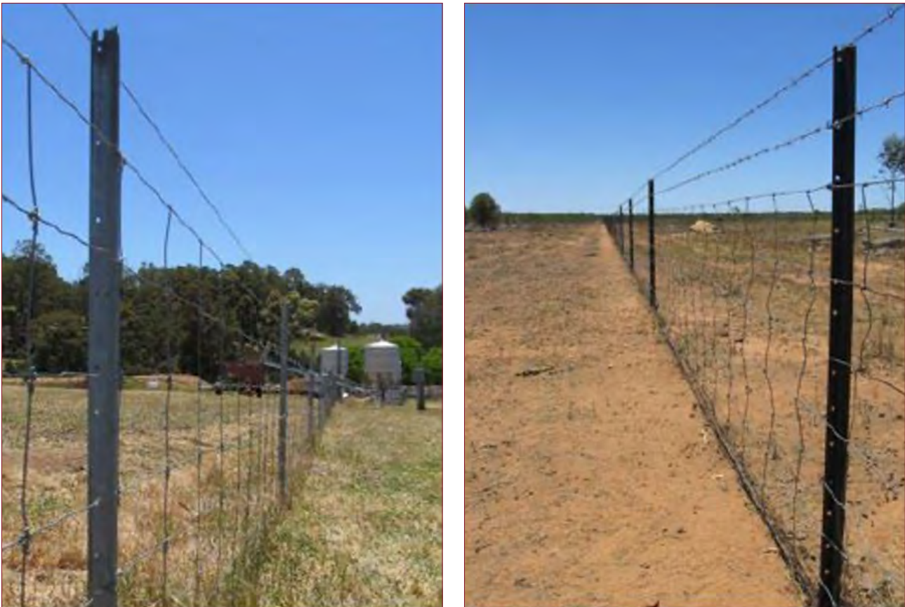
Figure 34: Examples of well-constructed ringlock fences
