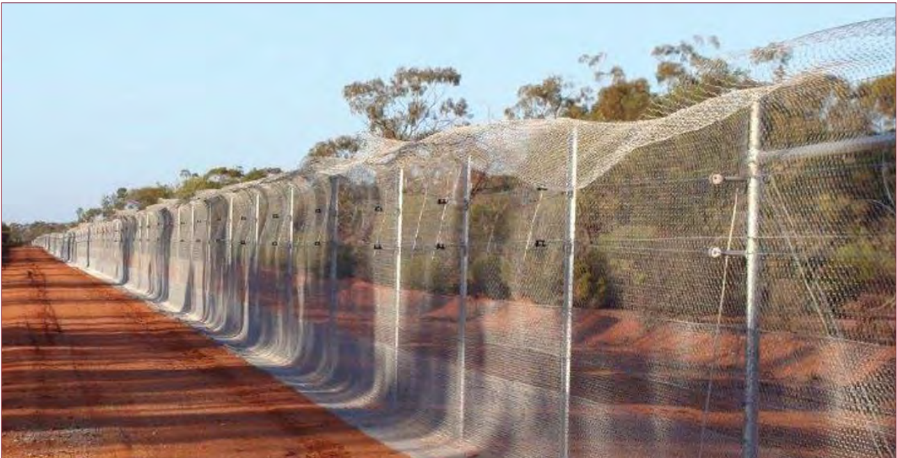
Figure 38: Example of an exclusion fence constructed with netting
