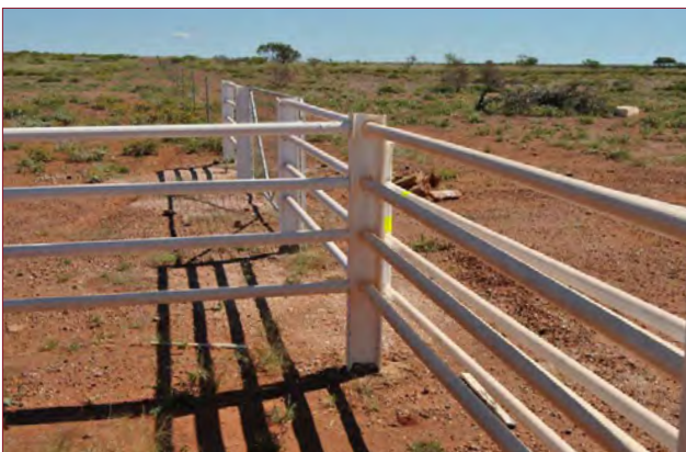
Figure 33: Fence strainers at a gate
