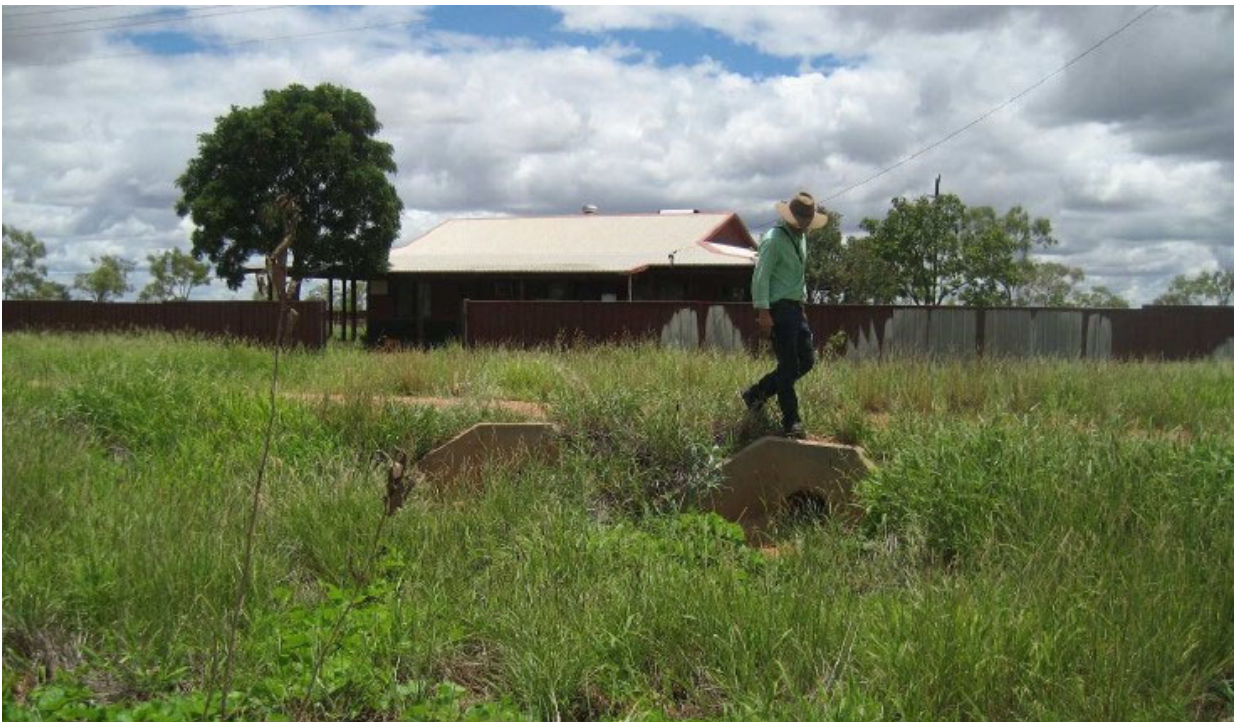
Figure 10 – Culvert on Colin Street between SL-Lot 40 and 50
