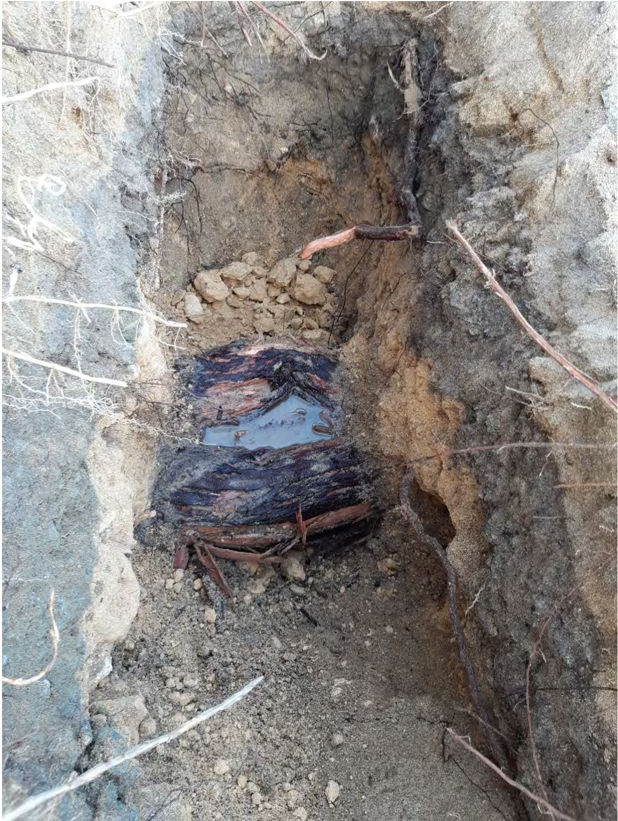
Tree root causing damage to Fern Rd and adjacent footpath located at Castledare between Cahill Court and Bungaree Rd
