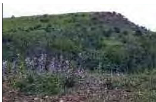
Figure 5: Existing flora on the range is fragmented (note erosion evident on the side slope).
