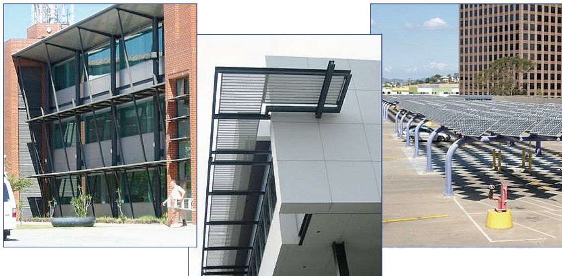
Figure 2: Examples of design solutions for reducing energy consumption through the use of passive shading controls, or through the use of active systems such as photo-voltaic arrays incorporated into car parking shade structures (which could be used to charge electric vehicles in the future).
