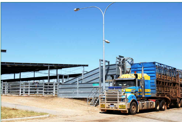
WAMIA facility in Precinct 1B (north B)
