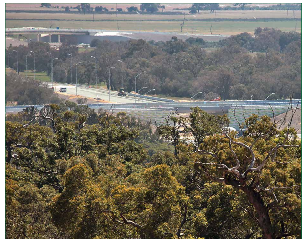
NorthLink under construction
