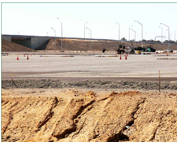
RTAA facility under construction in Muchea
