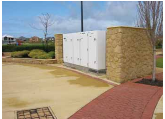
Figure 3 – A local park is used to provide a buffer to this wastewater pump station
