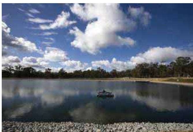
Figure 1 – Wastewater treatment plants provide essential services but from time to time may generate odour and need buffers to prevent land use conflict
