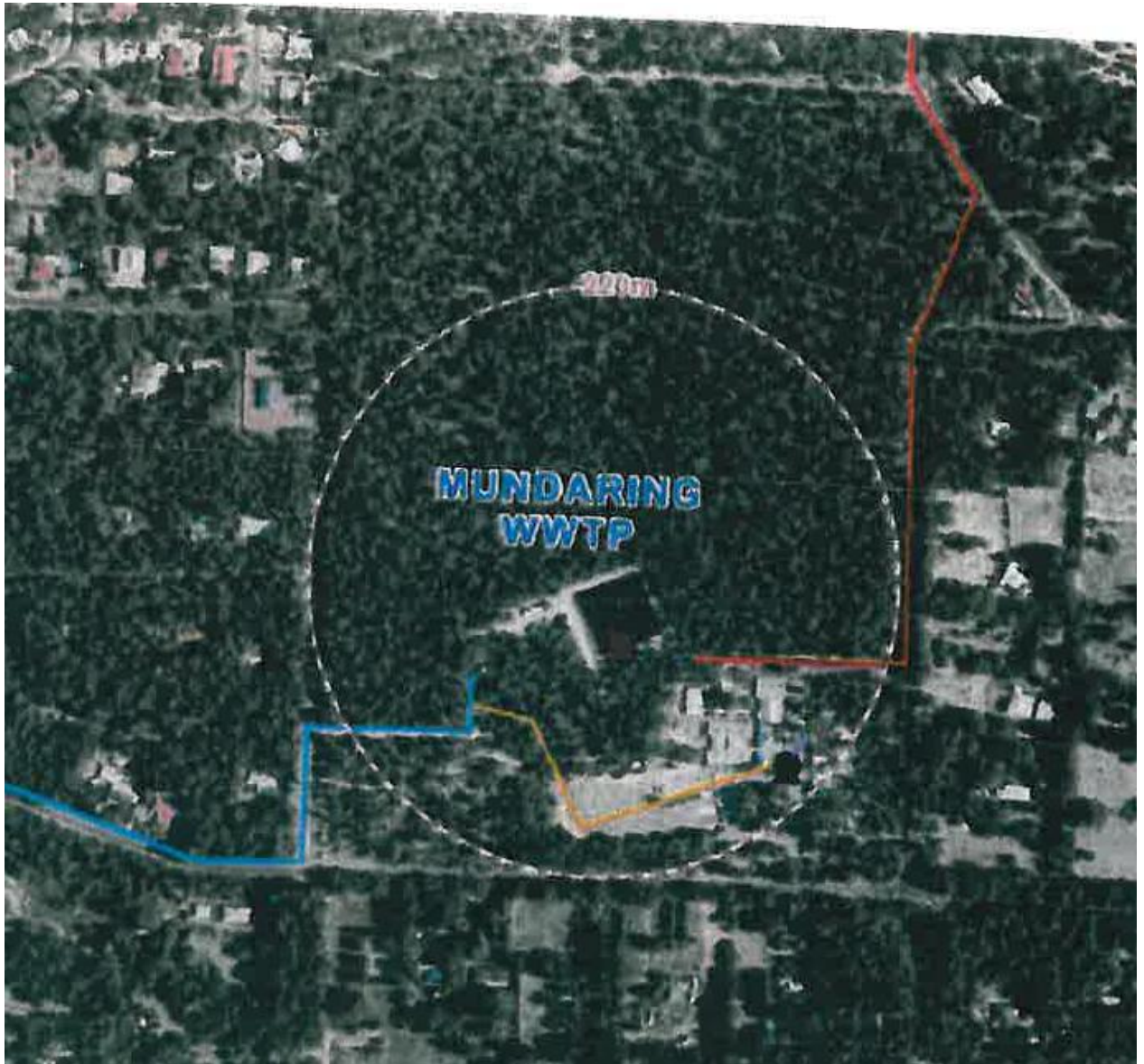
Figure 488: Mundaring Wastewater Treatment Plan odour buffer (source: Water Corporation)
