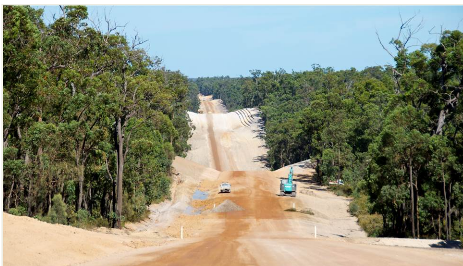
Mowen Road construction project
