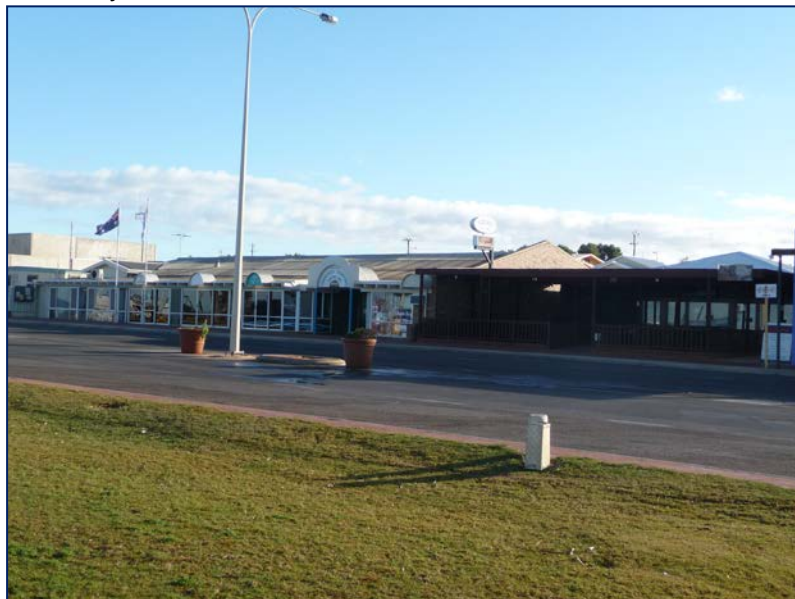
Shire Office : Knight Terrace
