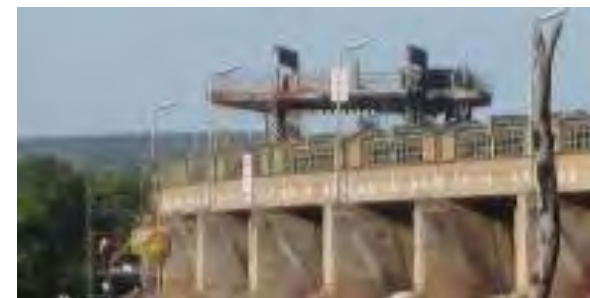
Annual maintenance on the diversion dam reduces capacity on the bridge crossing the Ord River, creating traffic impacts
