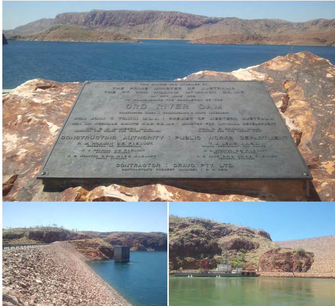
The Ord River Dam and hydroelectric power station are significant infrastructure assets, and also tourism attractions within Lake Argyle
