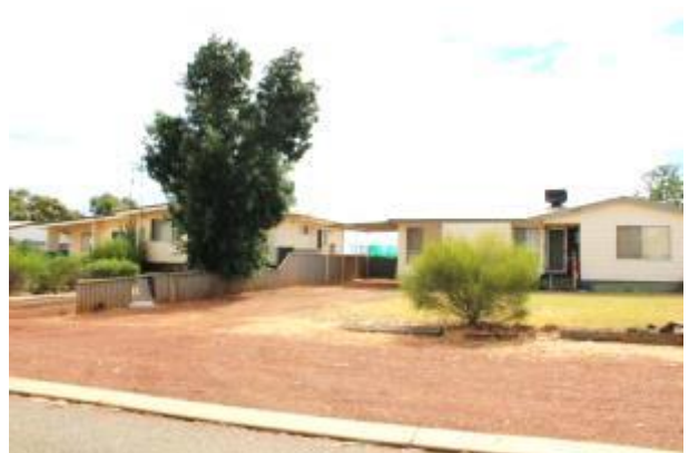
PICTURE 8 – OLDER COOROW HOUSING
