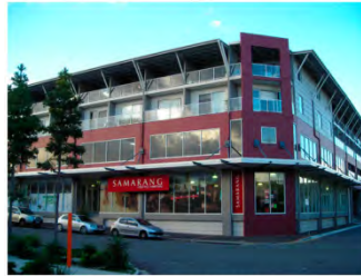
Furniture showroom with residential above
