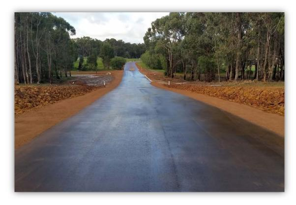
Figure 3 - Typical Rural Formation roadway with Scour Protection and Lowpoint Kerbing
