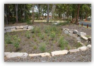
Typical sub catchment scale bioretention basin
