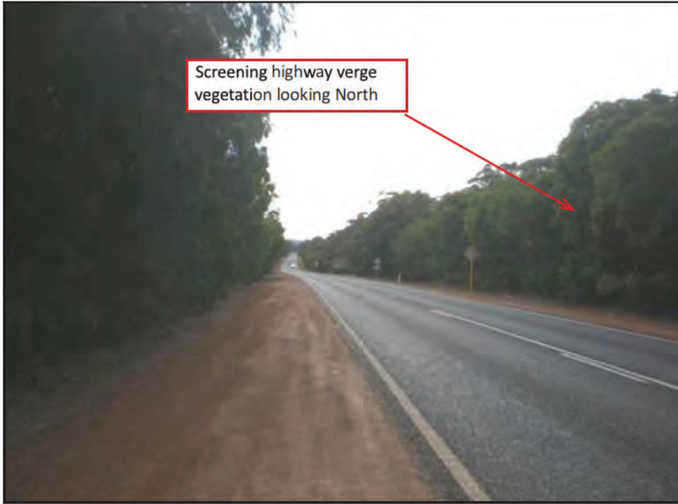
Image 1: View North along Bussell Hwy from the southern end of site showing the extent of existing screening verge vegetation to right of frame.
