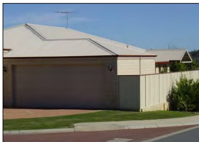
Photo 1: Unacceptable corner treatment
