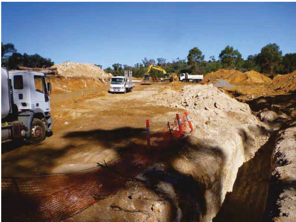
Photograph 6: Current development located nearby the site at the corner of McDonald Road and Fifty Road. Note the presence of shallow massive limestone
