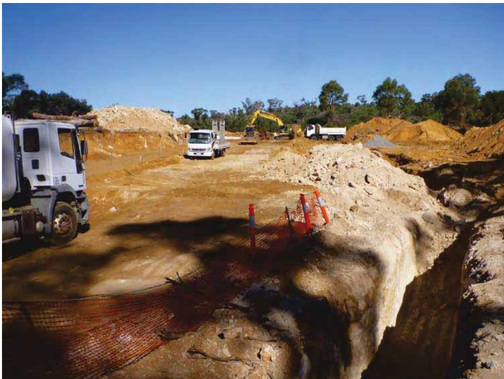
Photograph 6: Current development located nearby the site at the corner of McDonald Road and Fifty Road. Note the presence of shallow massive limestone
