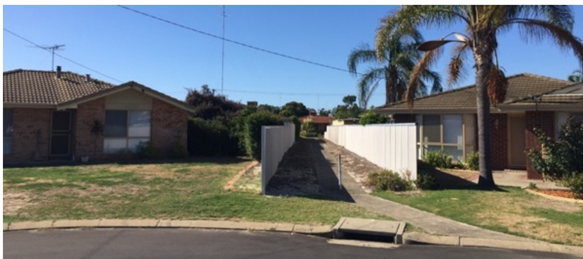
Photo 14: housing straddling a pedestrian access way on Hough Place, in the Residential / Mixed Use Precinct
