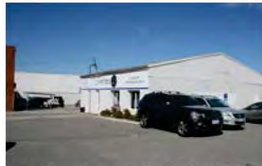
Parking areas on the south side provide minimal to no shelter.
