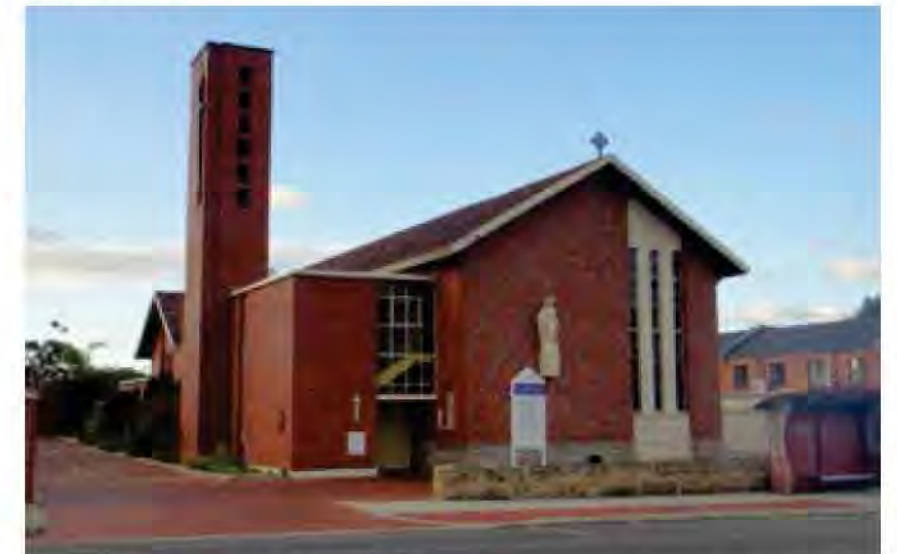
Our Lady of Victories Church - one of few heritage landmark buildings in the Centre.
