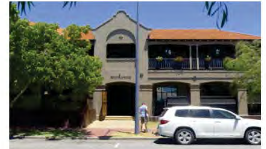
Wembley Hotel, the iconic building of the Wembley Centre and the centre's heart in the collective mind.
