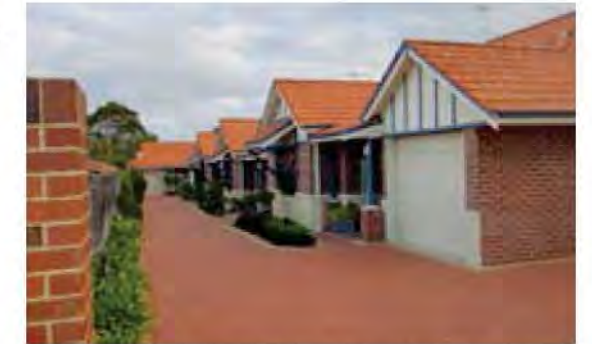
Strata title lots along Cambridge Street and Salvado Road with grouped dwellings on one lot.
