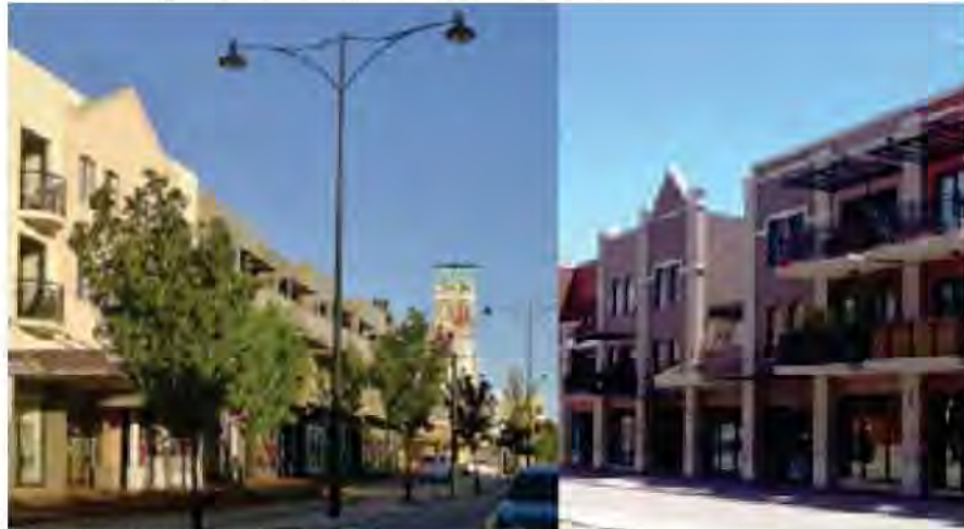
Examples of three storey street fronts
