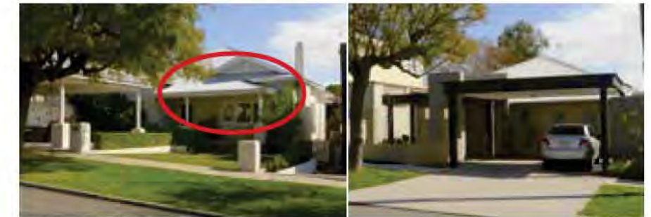
Characteristic overhanging roofs with shaded facades, in traditional and modern form
