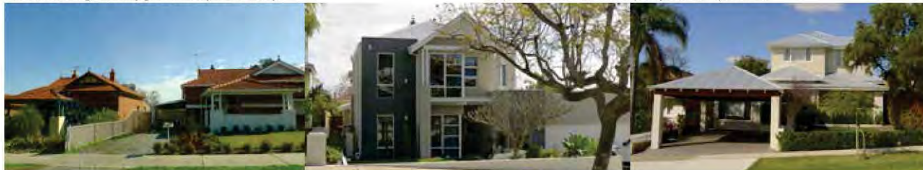
Traditional roof forms of single storey Wembley homes.....do not necessarily translate when applied to multi-storey buildings
