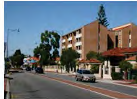
Existing tall buildings assist in orientation and way-finding in the town centre.
