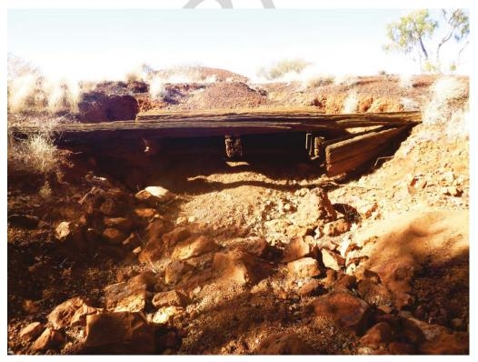
Plate 10: Off- site drainage culvert beneath former railway line
