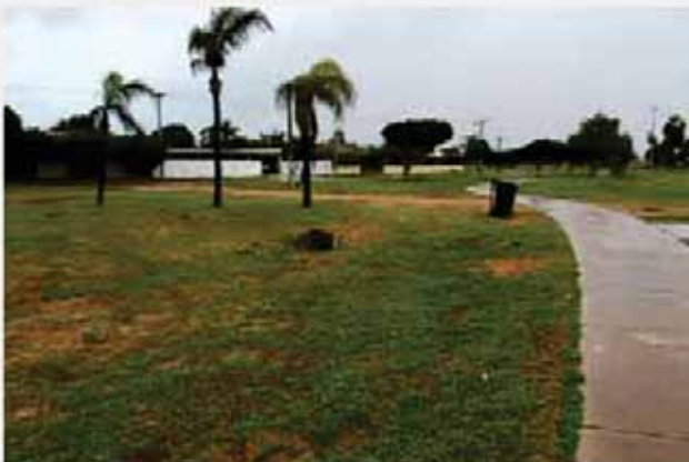
Existing drainage outlet within Structure Plan Area
