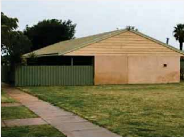
Existing building within GMF site
