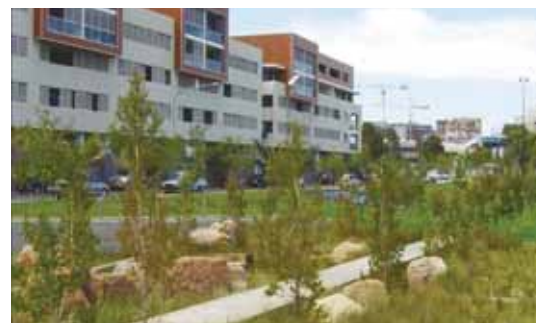
Figure 125: Low Impact Stormwater Design - Bioswales
