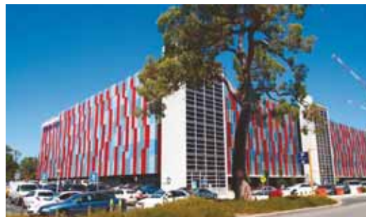
Figure 84: Parking Garage Screening (QEII, Nedlands)
