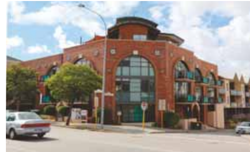
Figure 77: Landmark Corner (West Perth)
