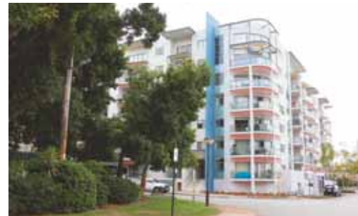
Figure 78: Landmark Corner (West Perth)
