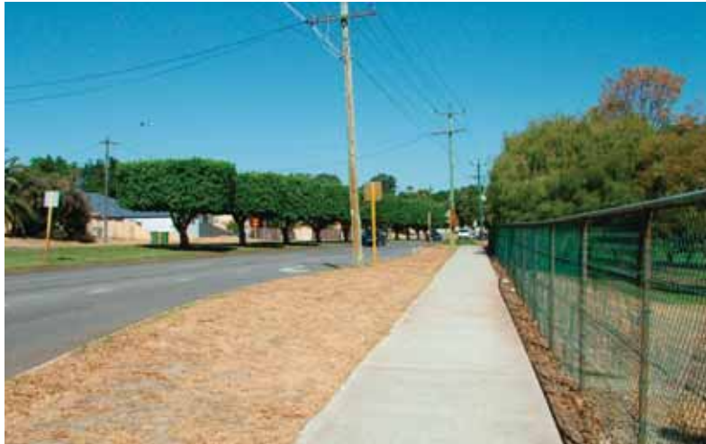
Figure 41 - Existing Broun Avenue
