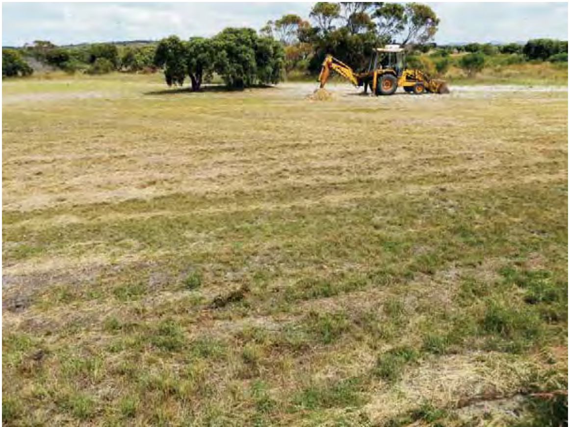
General view in the location of Hole 9
