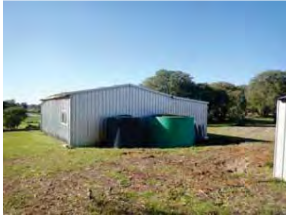
Photo location 26: existing water tanks and sheds within the site, looking north-east.
