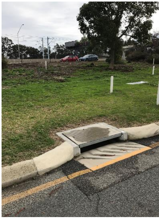
e) Existing stormwater side entry pit presents opportunity to retrofit as tree pit, providing both landscape, amenity and water quality treatment benefits
