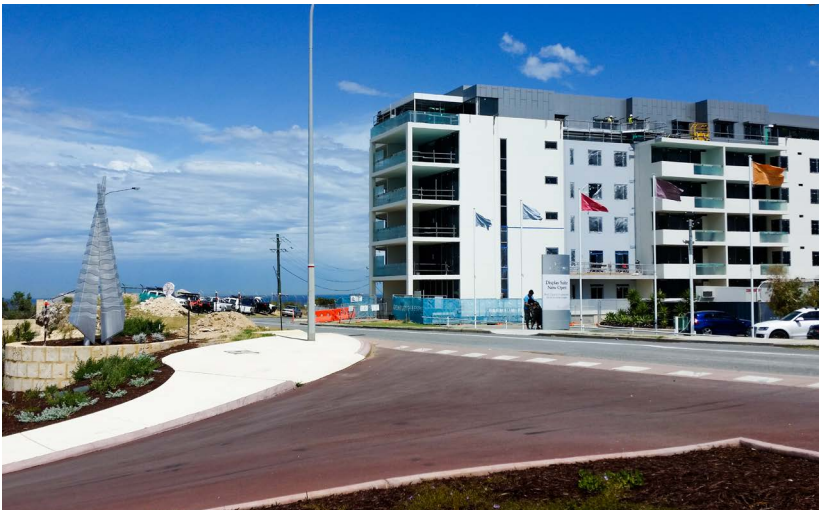
Taskers development on the northern side of McCabe Street, north-east of the Structure Plan Area
