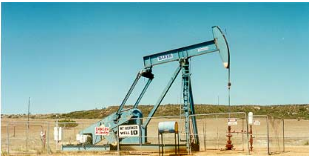
Plate 2: Oil production well, Mt Horner oilfield.
