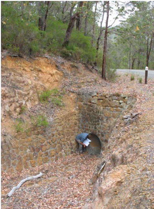
Photo 6 The constructed drain on the east of Bolganup Reservoir
