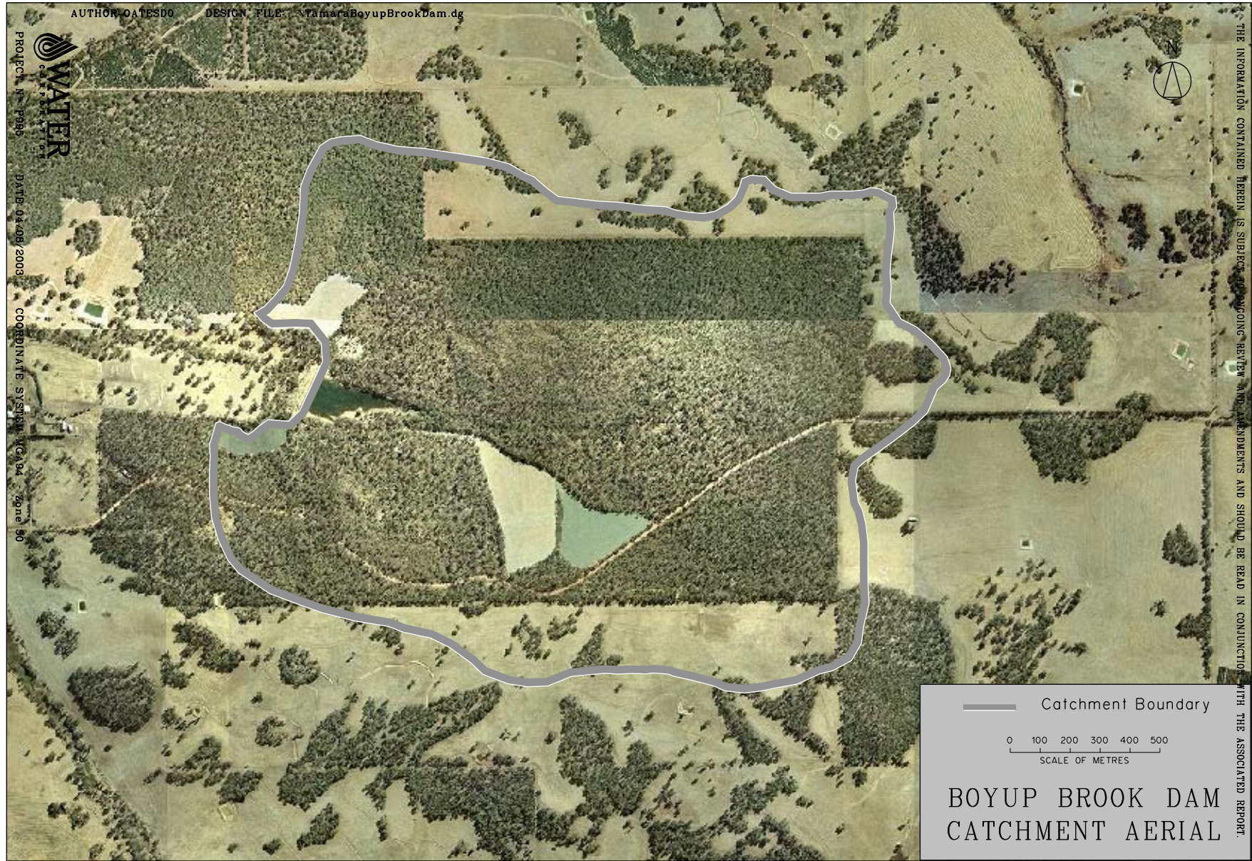
Photo 1 Boyup Brook Dam catchment aerial. The four bituminised areas are visible within the forested area.
