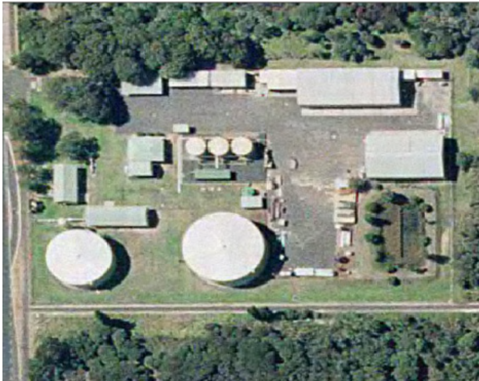
Figure B1 Water treatment plant 2 of Busselton Water (photo: Landgate)
